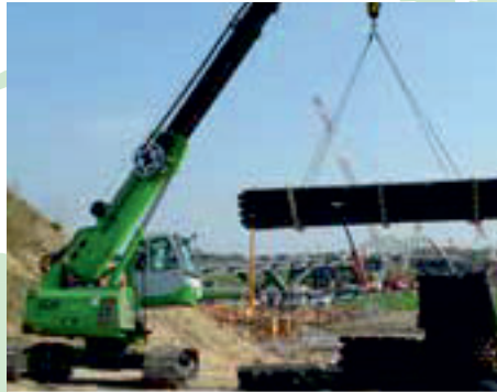
Civil engineering Tiefbau
