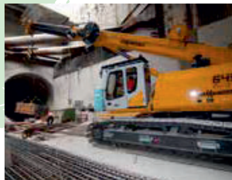
Tunnel construction Tunnelbau
